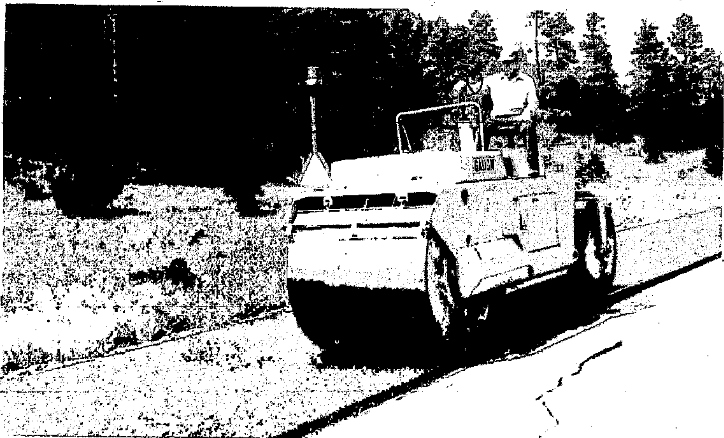
FLATTENING IT OUT is the job of steel roller operator Orlando Lucero. The hot asphalt (temperature 275 degrees) goes through the
