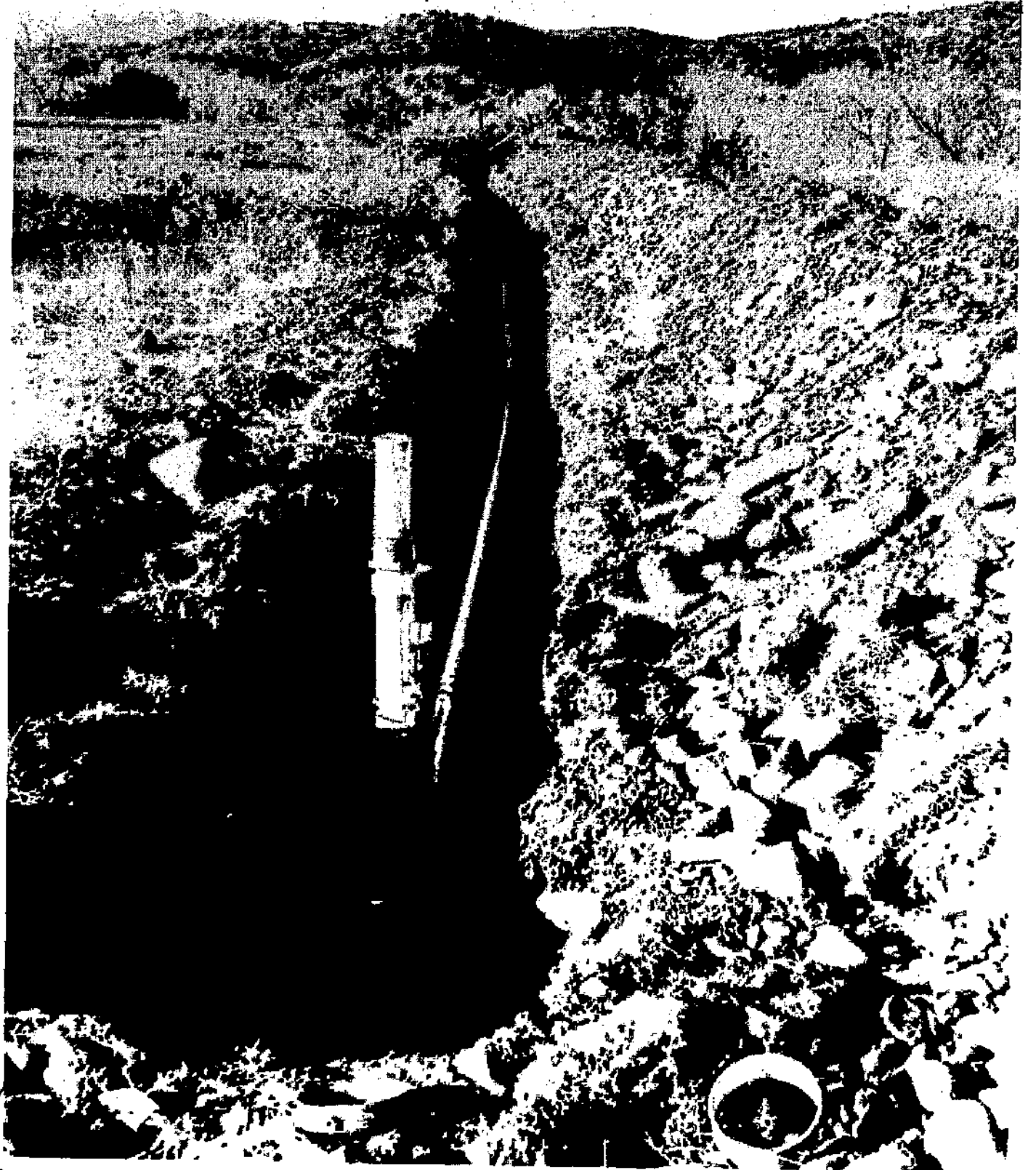
NEARLY A MILE OF PLASTIC pipe completes the irrigation pipeline project. The rocky material on the banks is the porous material through which the water drained when the old irrigation ditch was in use.
