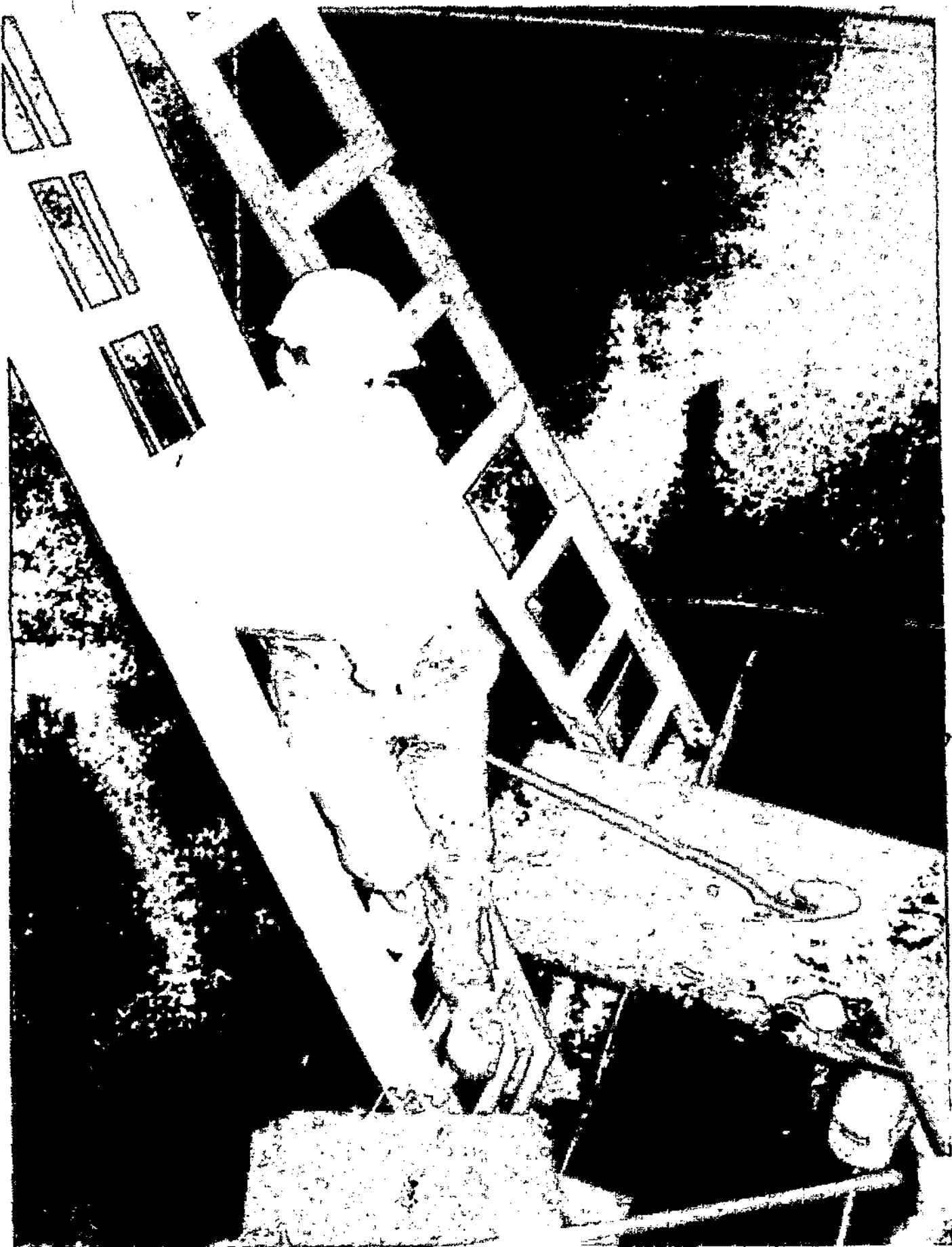
JUST A PAUSE in filling the treatment tank at the Upper Canyon water treatment plant with new filter material. Elmer Schalles of Interwest Limited from Albuquerque, the contractors who have been repairing the tank since April, rests during the last step of the repairs. When back on line this week, the plant will be capable of treating over 400,000 gallons a day, a big jump from the 200,000 gallons it was handling before repairs.
