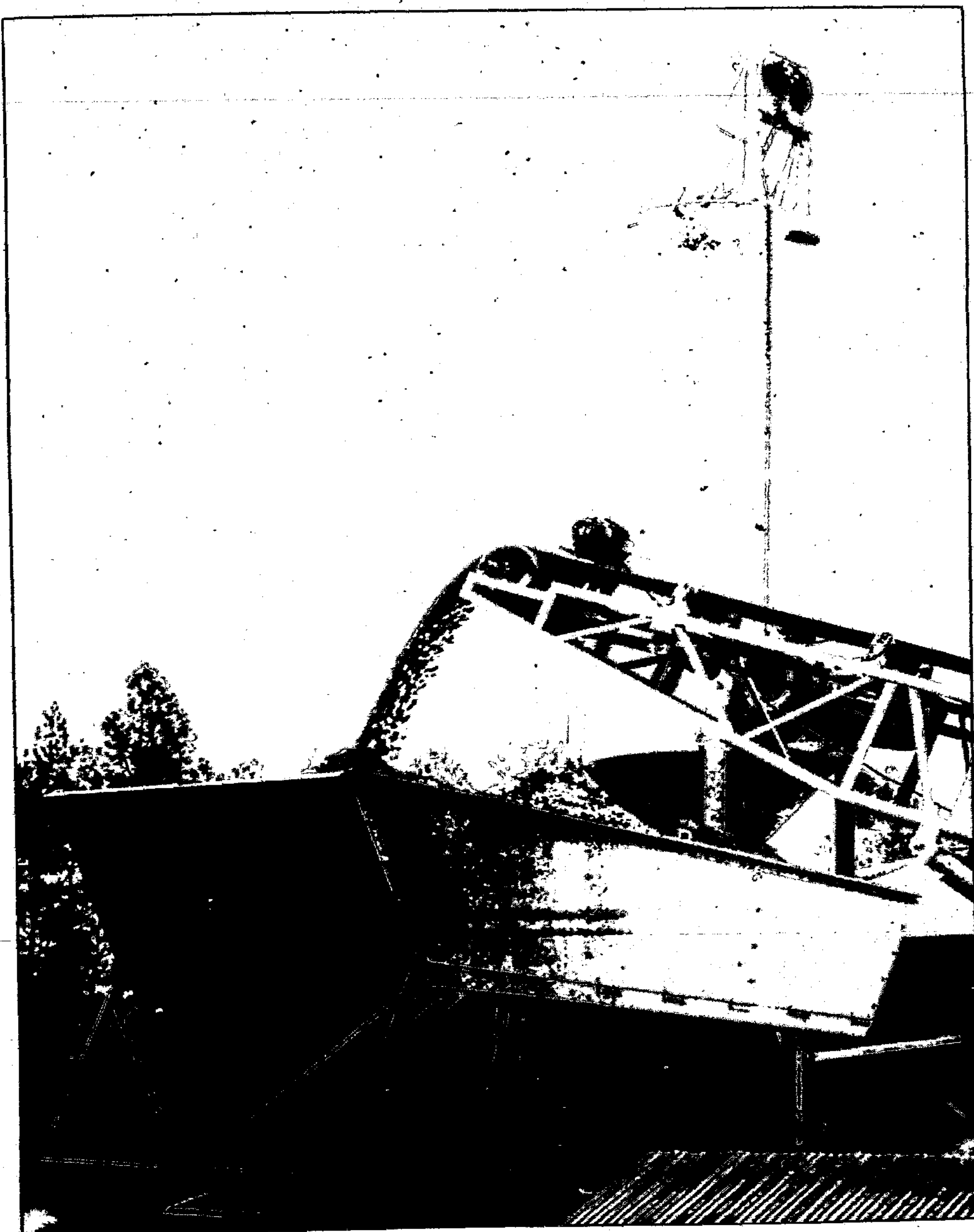
A conveyor belt moves materials to the Grindstone Canyon dam from huge piles of aggregate. Concrete laying at the roller-compacted process dam continues 20 hours a day.
