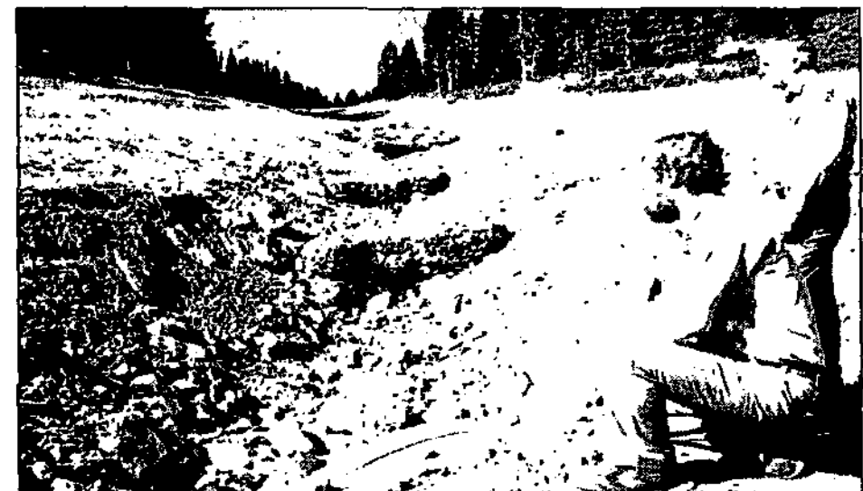
Foresters Sam Tobias, kneeling, and Jerry Hawkes, survey drainage improvements at Ski Apache in an area cut by a 15-foot deep gully in flooding last year. A culvert (in the foreground) has been added, as well as gabion baskets full of rocks to slow the water flow and catch silt, and mesh mats to encourage the growth of vegetation.
