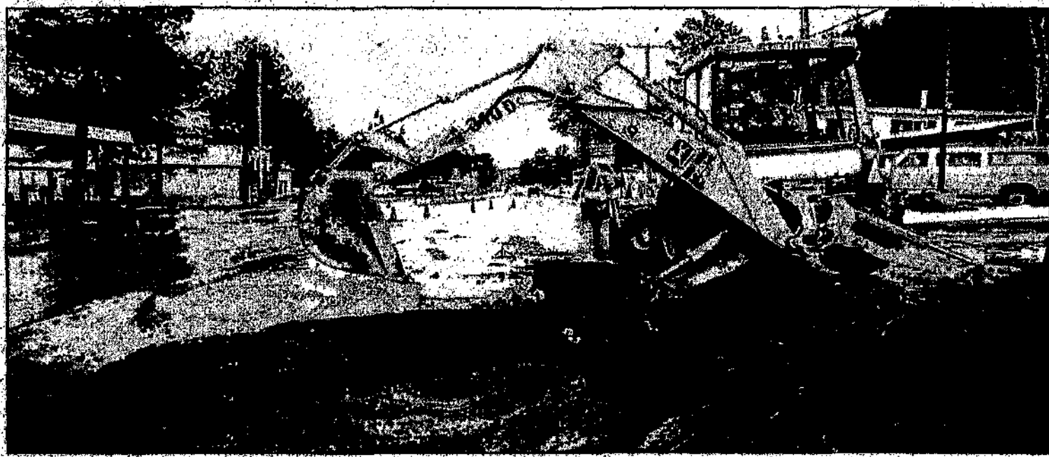
A Ruidoso village employee last week directs a hydraulic claw into a man-made crater on Sudderth Drive while trying to reach a broken six-inch water main.
