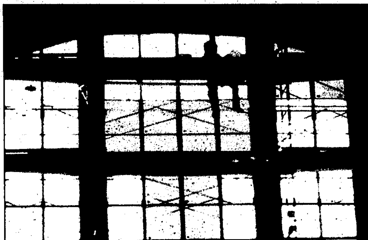
Shining like a beacon — a night time view of the church, above, shown with the all-new outdoor lighting. Below, removal of the old plexiglass panels to prepare for the new unbreakable fiberglass reinforced with copolymer plastic glass.
